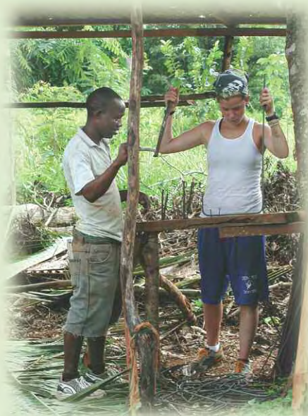
Kendra Benson and a construction worker bend rebar at Kisarawe Lutheran Jr. Seminary.
